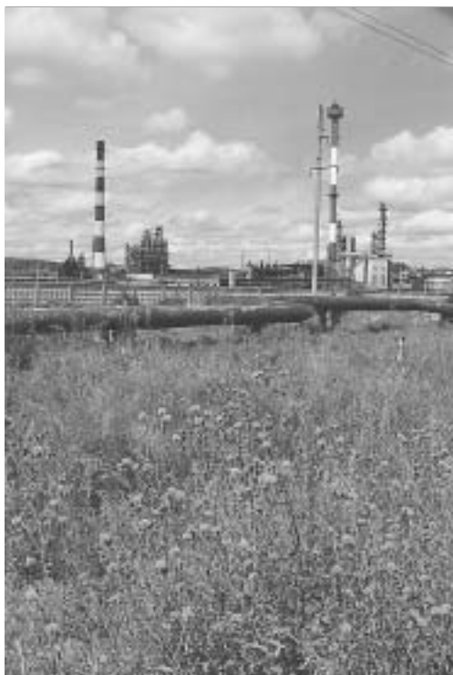
Photo 7. A Corner of Rosneft Oil Refinery Plant, Komsomolsk-na-Amure (Credit : H. M. 2003)
