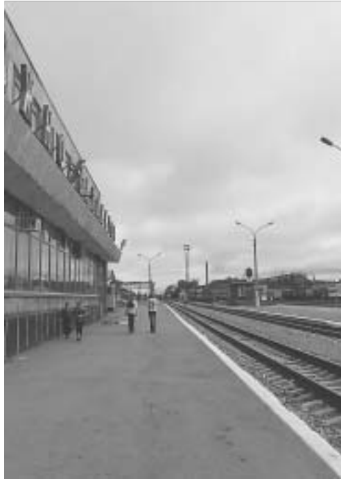
Photo 1. Railway Station of Yuzhno-Sakhalinsk, the Rail Being the Japanese Narrow Gauge, Sakhalin (Credit : H. M. 2002)
