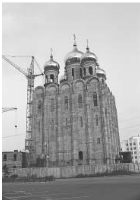
Photo 12. Big Church under Construction, Magadan (Credit : H. M. 2003)
