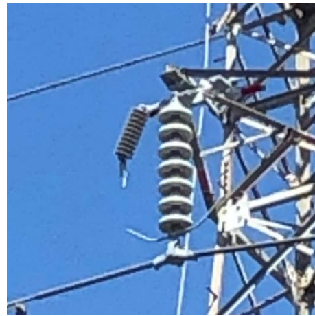
(b) Arcing-horn type metal-oxide surge arrester
