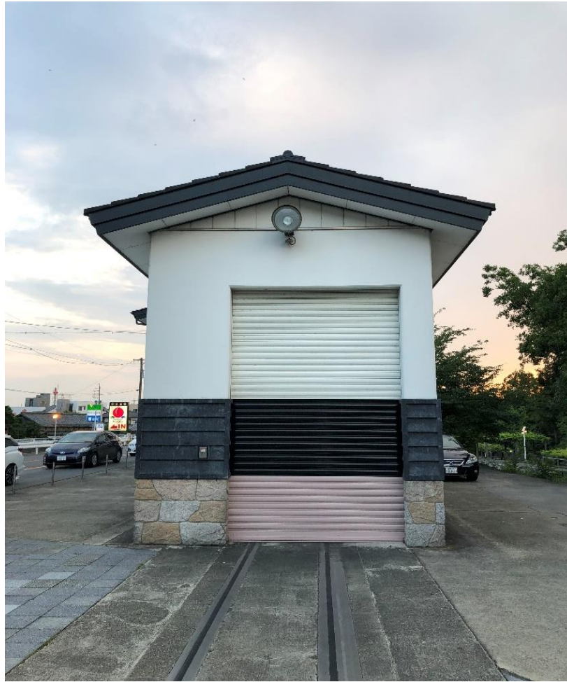
Figure 4.7. Flood Control Gates and Warning System for Flood Prevention in Gifu
