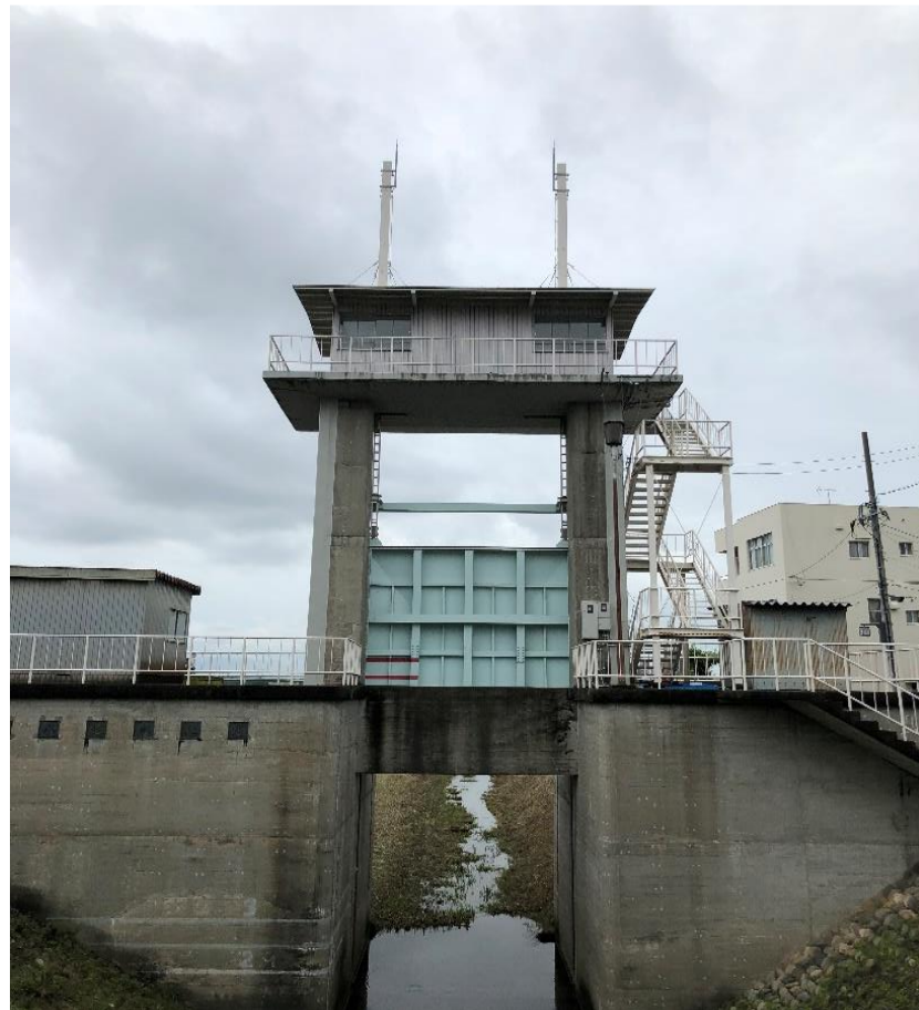
Figure 4.6. Flood Control Gates for Flood Prevention in Gifu (Source: Author, from July 2019 fieldwork)
