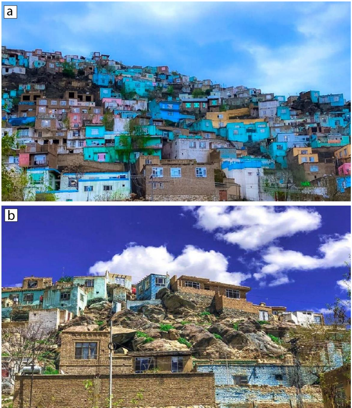
Figure 5.11: Houses on the slop of mountain in Kabul City. a) Homes, seemingly built on top of the next. b) Houses on the south slope of Koh-i-Asmai Mountain (Photos by Mohamad Hamid Hamdard).
