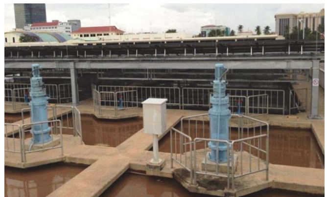
Fig. 4 Flocculation basin
