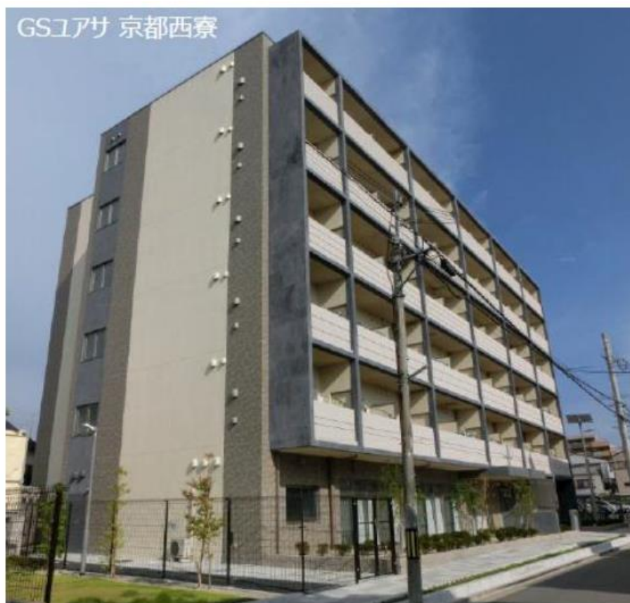
Fig. 5.10 An exterior view of the field test facility.
