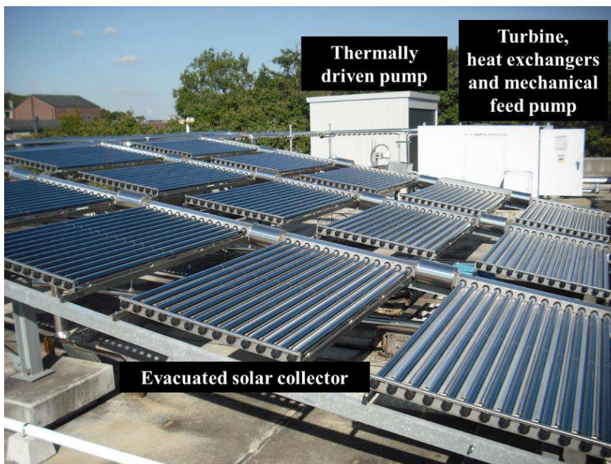
Figure 3.1. The outlook of supercritical CO 2 solar Rankine cycle system.
